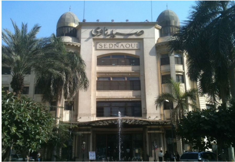
Figure 26. Photograph of Sednaoui department store, Cairo, 2013, by author.
